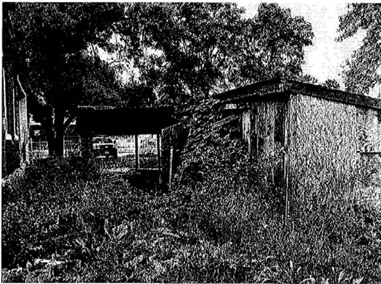
North Face Carport
