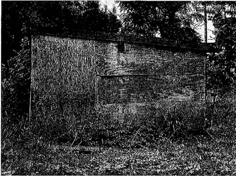
West Face Carport
