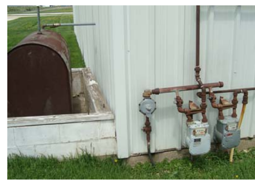
BOX HANGAR (TYPE A) PHOTOS
