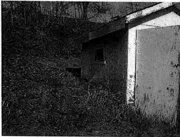
Shed South Face
