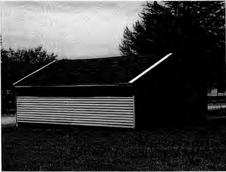
Garage/ Garage Roof
