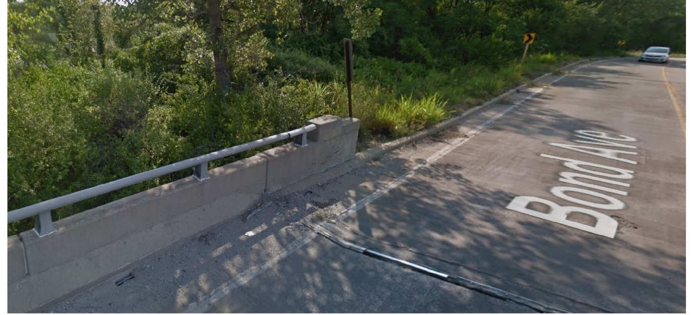
EAST ABUTMENT NORTH WINGWALL
