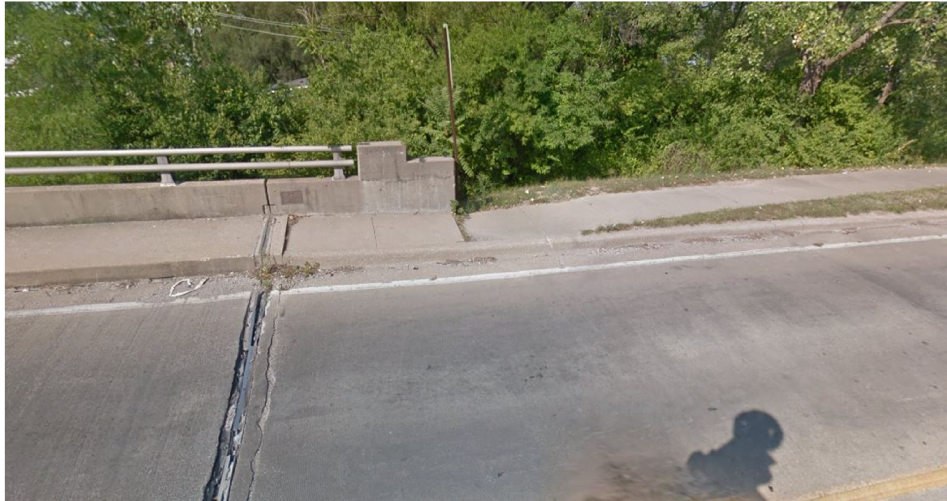
WEST ABUTMENT SOUTH WINGWALL
