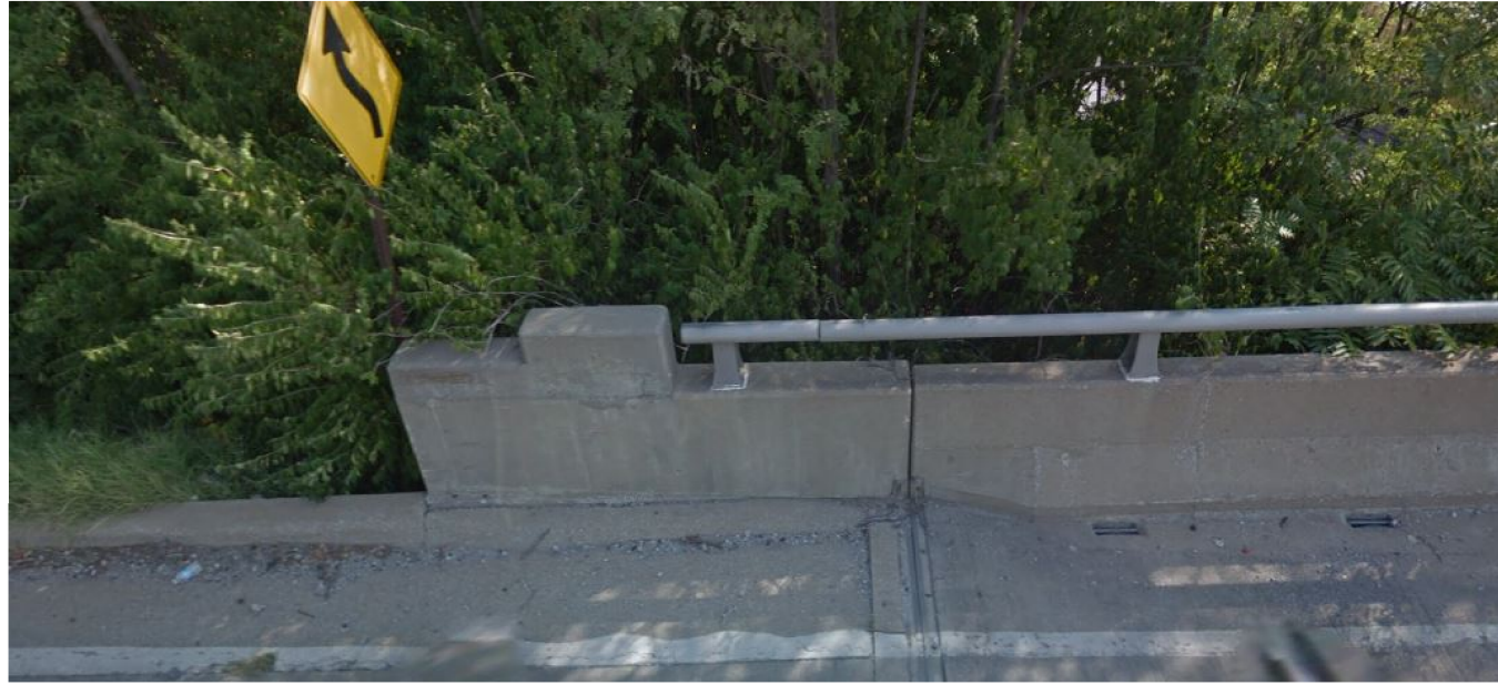
WEST ABUTMENT NORTH WINGWALL
