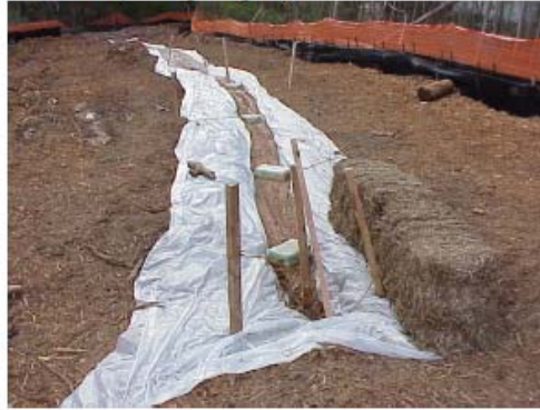
6) Ready for pumping
