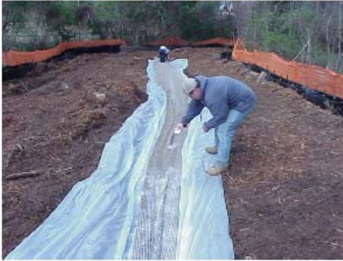
5) Apply Silt Stop (downstream end)
