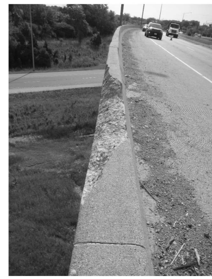
PARAPET DAMAGE
