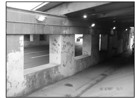
EXISTING LIGHTING: PIER 1 (Looking Southeast)
