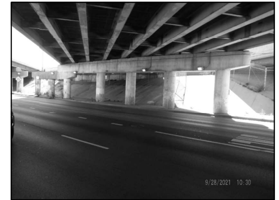
EXISTING LIGHTING PIER 2 (Looking Southeast)
