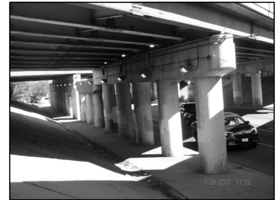
EXISTING LIGHTING PIER 1 (Looking Southeast)
