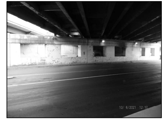
EXISTING LIGHTING: PIER 2 (Looking Southeast)
