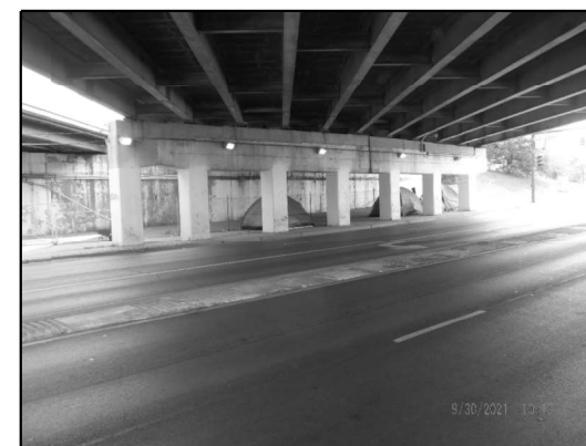
EXISTING LIGHTING: PIER 1 (Looking Southeast)
