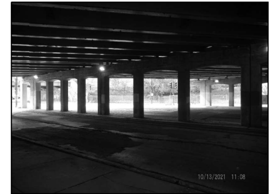
EXISTING LIGHTING: PIER 1 (Looking Southwest)
