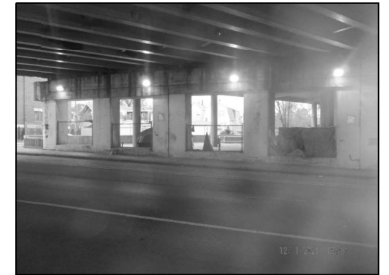
EXISTING LIGHTING: PIER 2 (Looking Southeast)
