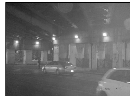
EXISTING LIGHTING: PIER 1 (Looking Southeast)
