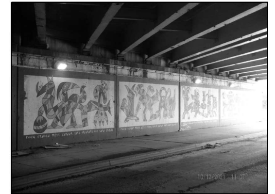
EXISTING LIGHTING: EAST ABUTMENT (Looking Southeast)
