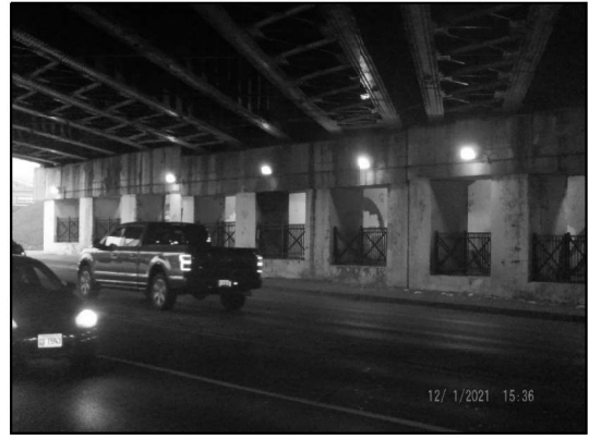
EXISTING LIGHTING: WEST ABUTMENT (Looking Northwest)
