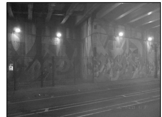
EXISTING LIGHTING: EAST ABUTMENT (Looking Southeast)
