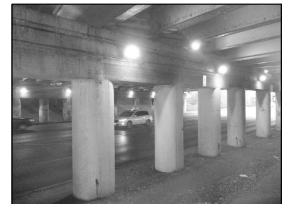
EXISTING LIGHTING: PIER 1 (Looking Northeast)
