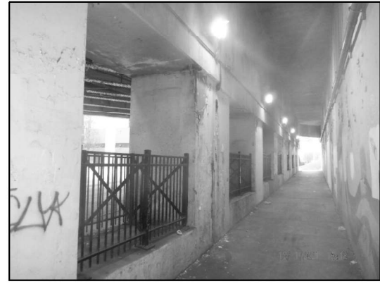
EXISTING LIGHTING: WEST ABUTMENT (Looking Southwest)
