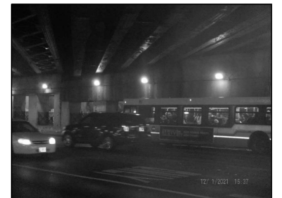
EXISTING LIGHTING: WEST ABUTMENT (Looking Northwest)
