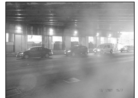
EXISTING LIGHTING: PIER 1 (Looking Southwest)
