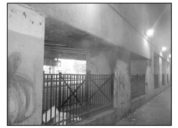
EXISTING LIGHTING: WEST ABUTMENT (Looking Southwest)
