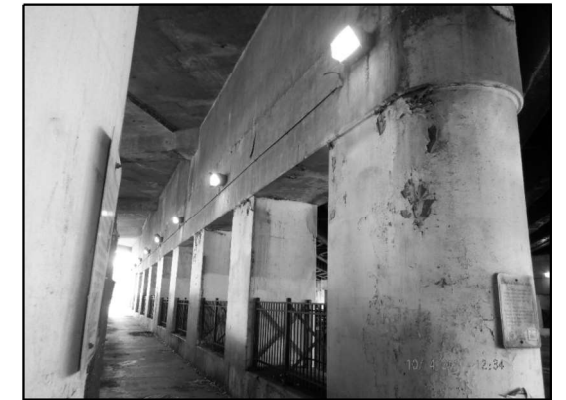
EXISTING LIGHTING: PIER 1 (Looking Northeast)
