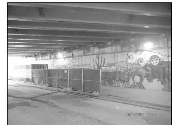
EXISTING LIGHTING: WEST ABUTMENT (Looking Northwest)
