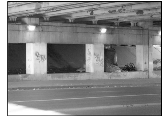
EXISTING LIGHTING: PIER 2 (Looking Northwest)
