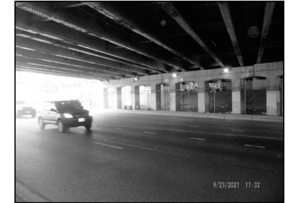
EXISTING LIGHTING: PIER 2 (Looking Northwest)
