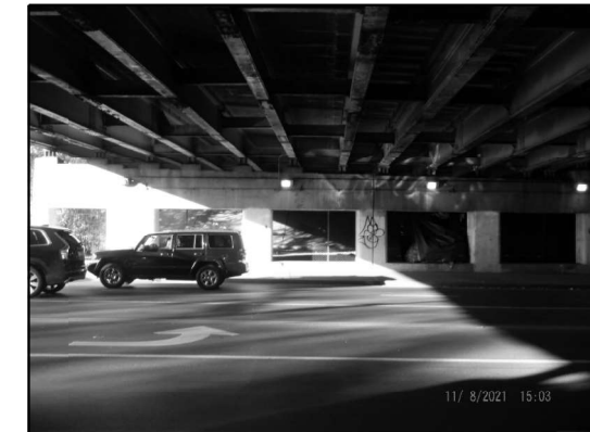
EXISTING LIGHTING: PIER 2 (Looking Northeast)
