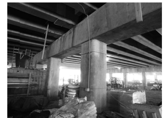
PIER 1 (Looking Northwest)
