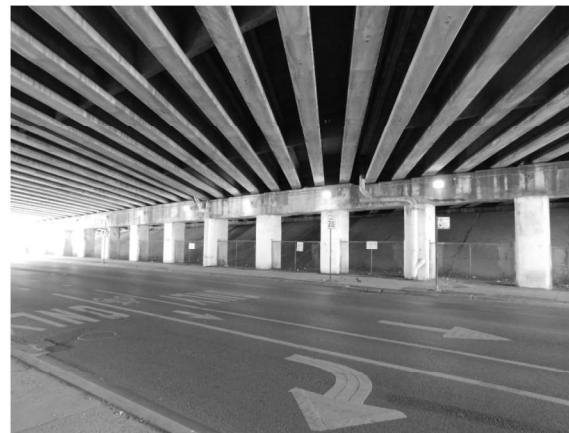
PIER 24 (Looking North)
