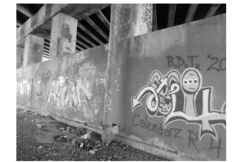
PIER 10 (Looking Northwest)
