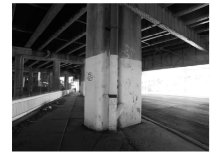
PIER 19 - EAST END (Looking Northeast)
