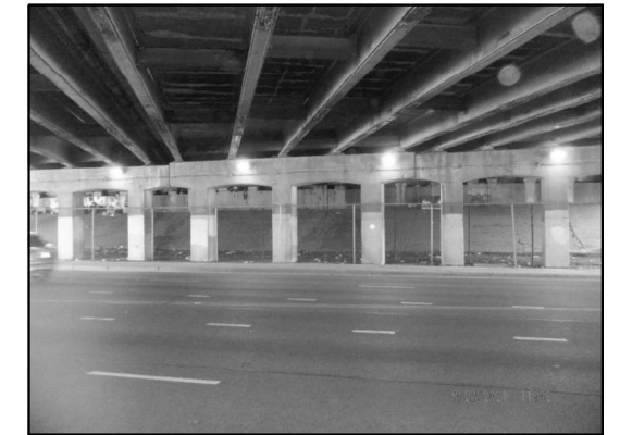
EXISTING LIGHTING: PIER 2 (Looking Northwest)
