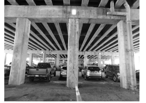
PIER 5 (Looking South)
