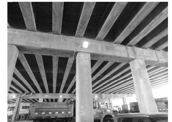
PIER 4 (Looking South)
