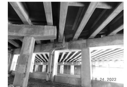
PIER 23 - EAST END (Looking North)
