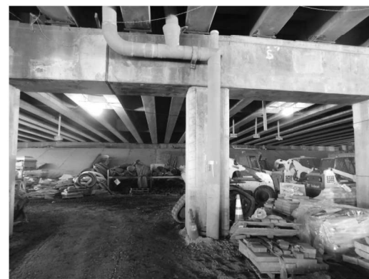
PIER 1 - EAST END (Looking South)
