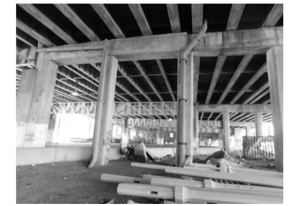
PIER 15 (Looking North)
