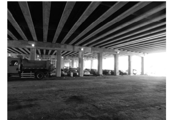
PIER 4 (Looking Northeast)
