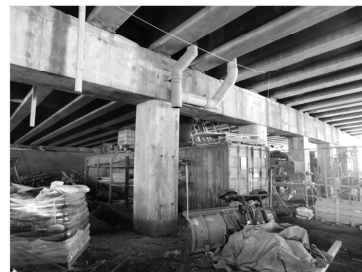
PIER 1 - WEST END (Looking Southwest)
