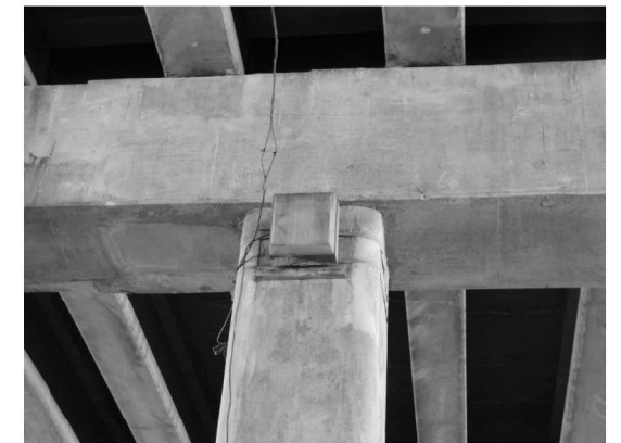
PIER 7 (Looking North)
