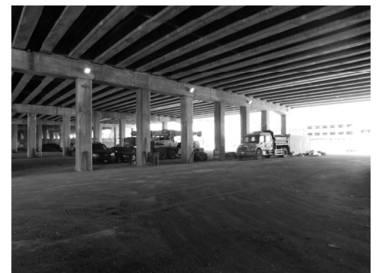
PIER 6 (Looking Northeast)
