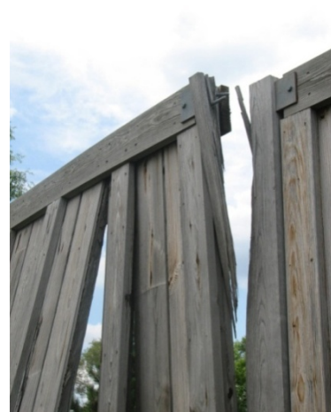
Photo 18. Side View of Damaged Panel (NAW 5) Photo 19. Failed Connection (NAW 5)
