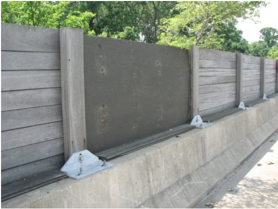
Photo 13. Temporary Repair Using Painted Plywood (NAW 3)
