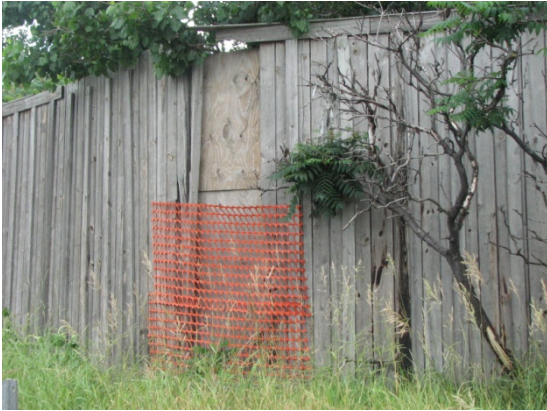
Photo 1. Plywood Repair (NAW 1)
