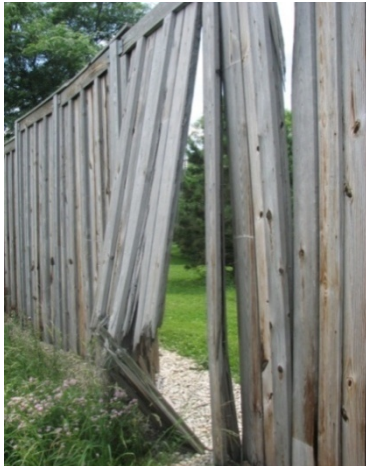
Photo 18. Side View of Damaged Panel (NAW 5) Photo 19. Failed Connection (NAW 5)
