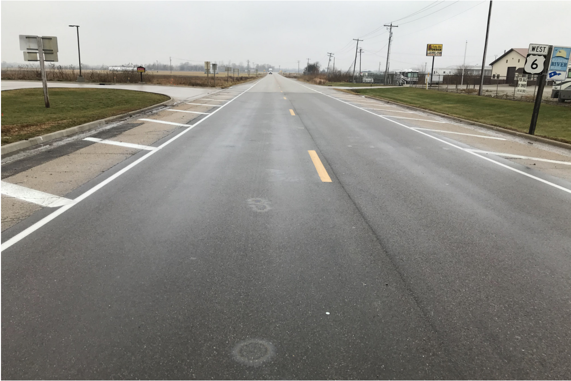
US RT 6 - Looking West
