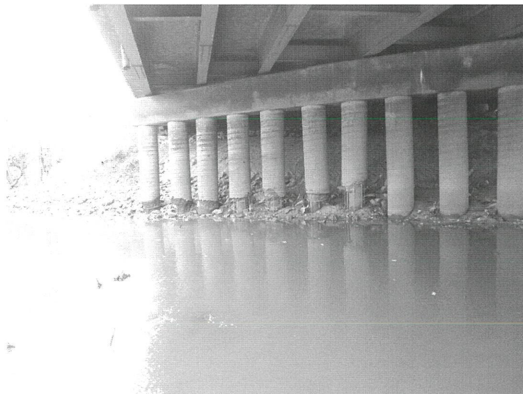
EAST PIER - LOOKING EAST
