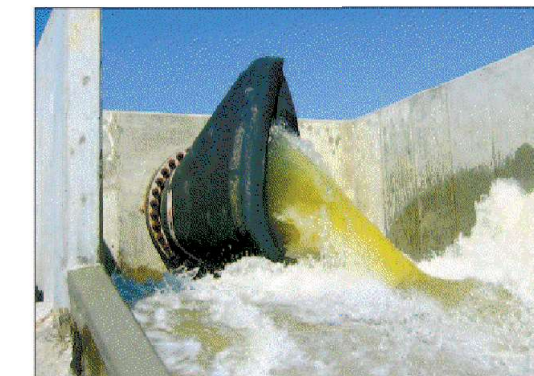
The increased driving head of a TF-1 Check Valve (or equivalent) improves flow capacity.
