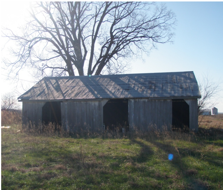
BUILDING 1: WOOD STORAGE BUILDING
