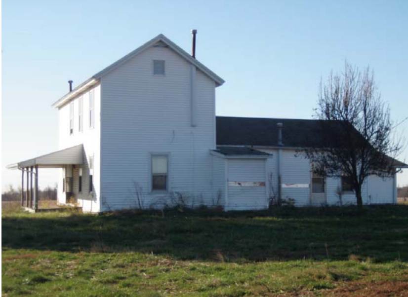
BUILDING 7: TWO STORY RESIDENCE
