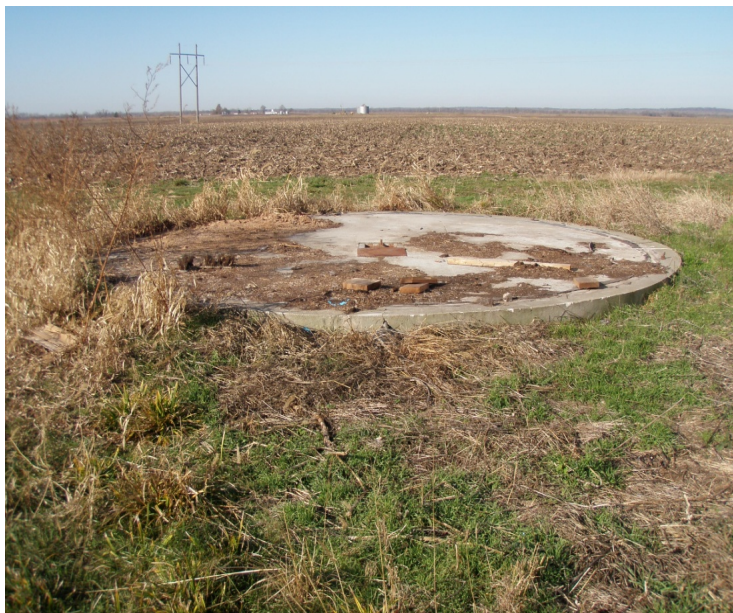
CONCRETE FOUNDATION FOR GRAIN BIN
