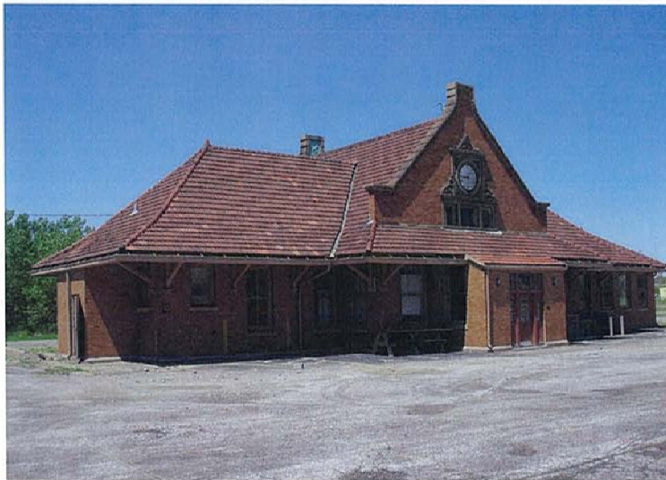
South Face/ Roof
