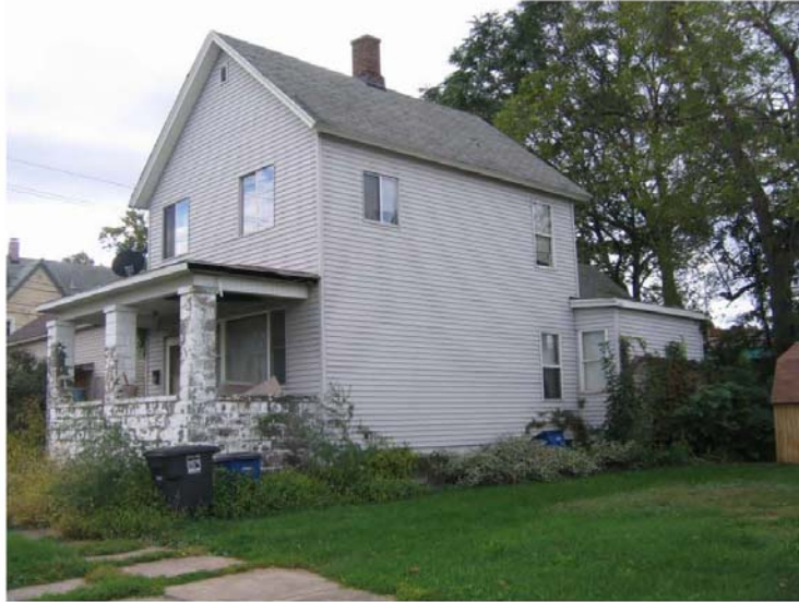
North Face/ Roof
