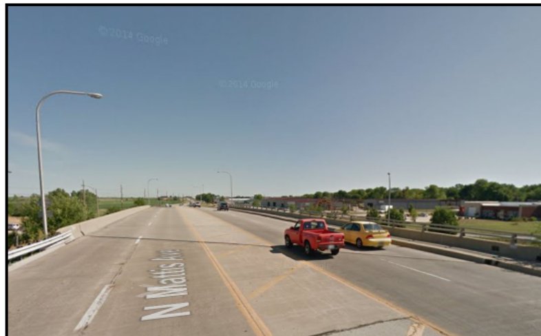
Exhibit 2: Existing N. Mattis Avenue over I-74
