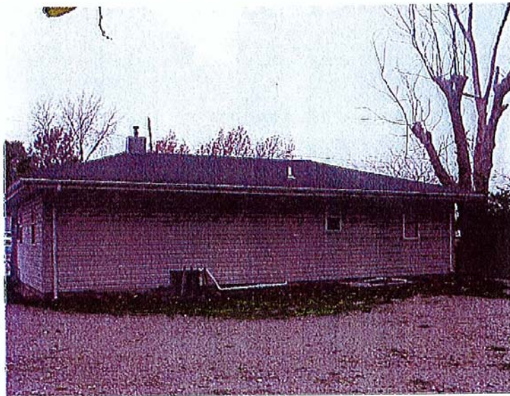
Rear, North Side of Building
