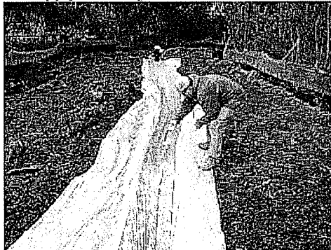
5) Apply Silt Stop (downstream end)
