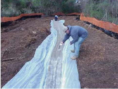
5) Apply Silt Stop (downstream end)
