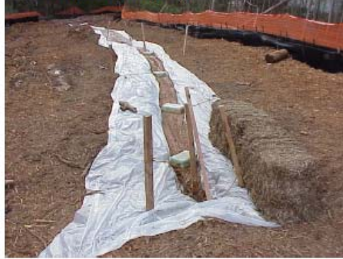
6) Ready for pumping
