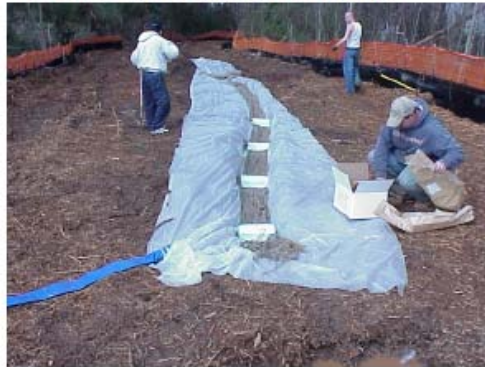
4) Place Floc Logs (upstream end)
