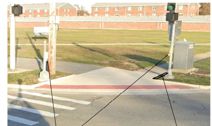
NORTH EAST CORNER
