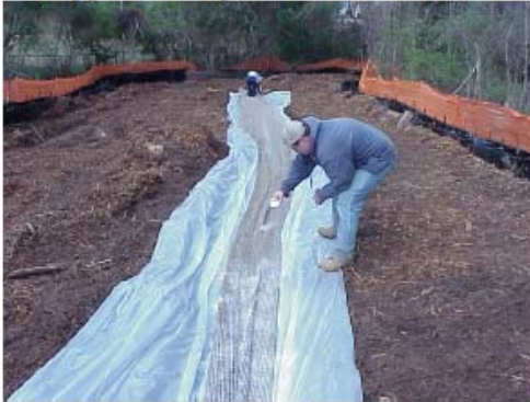
5) Apply Silt Stop (downstream end)
