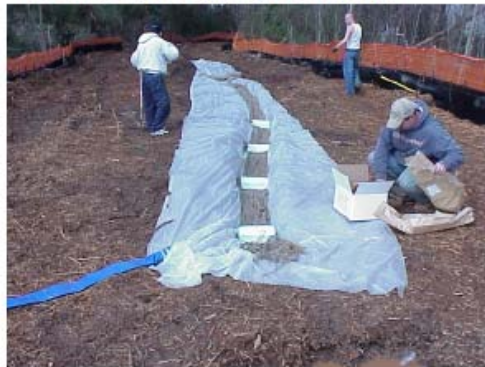
4) Place Floc Logs (upstream end)
