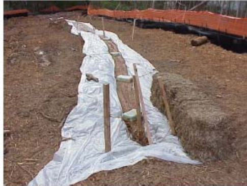
6) Ready for pumping
