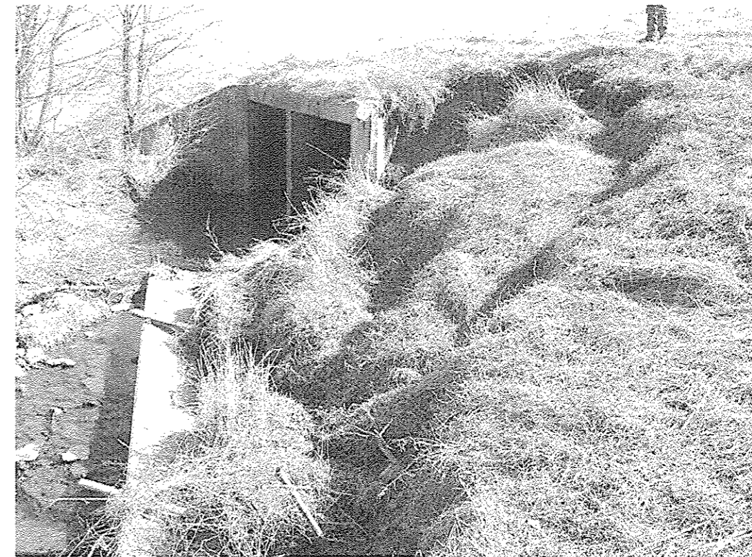
EXISTING CONDITIONS - SN 069-2004
