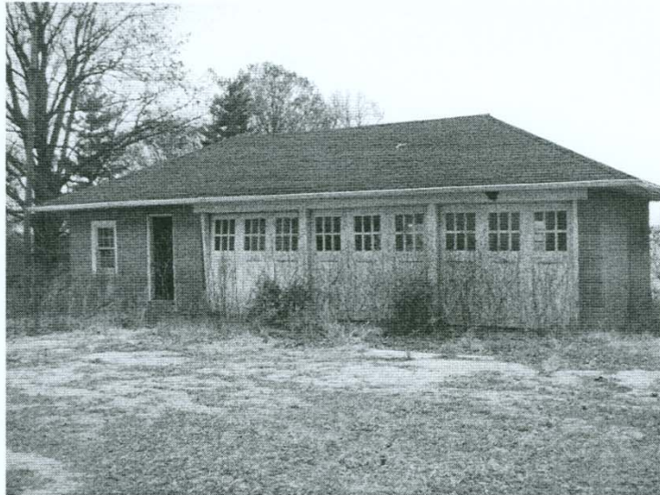
BUILDING # 2: SHOP BUILDING
