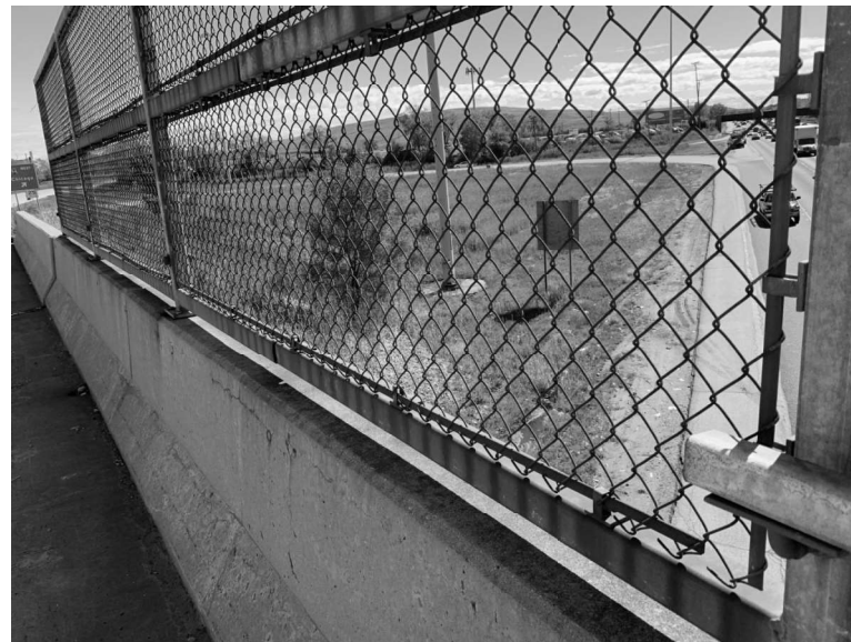
MISSING HANDRAIL
