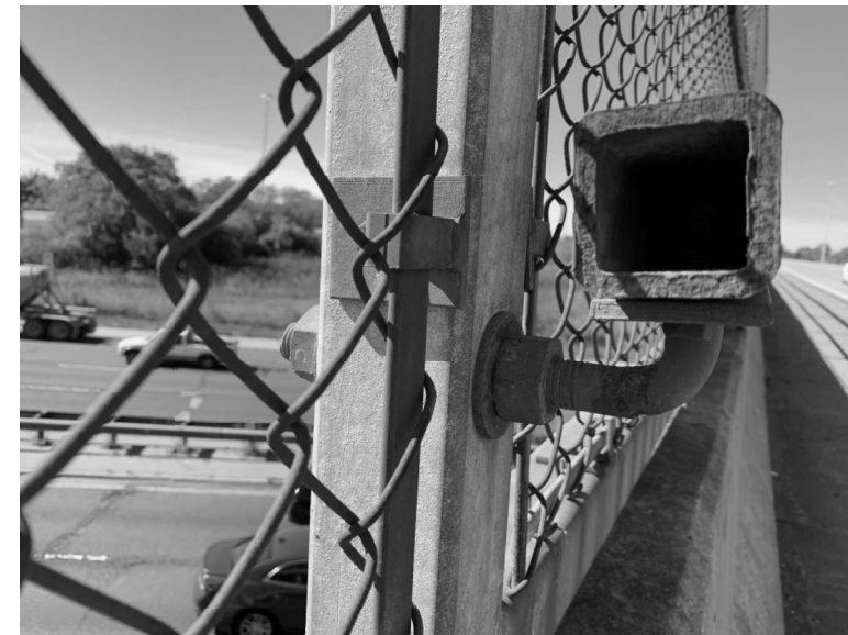
HANDRAIL ATTACHMENT DETAIL
