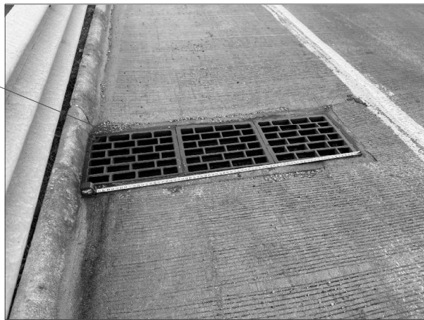
PHOTO OF EXISTING SHOULDER INLET ALONG CURB ON NORTH APPROACHES
