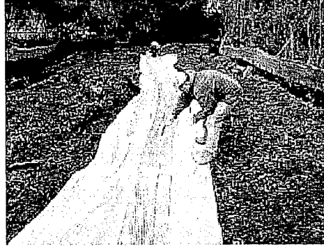
5) Apply Silt Stop (downstream end)
