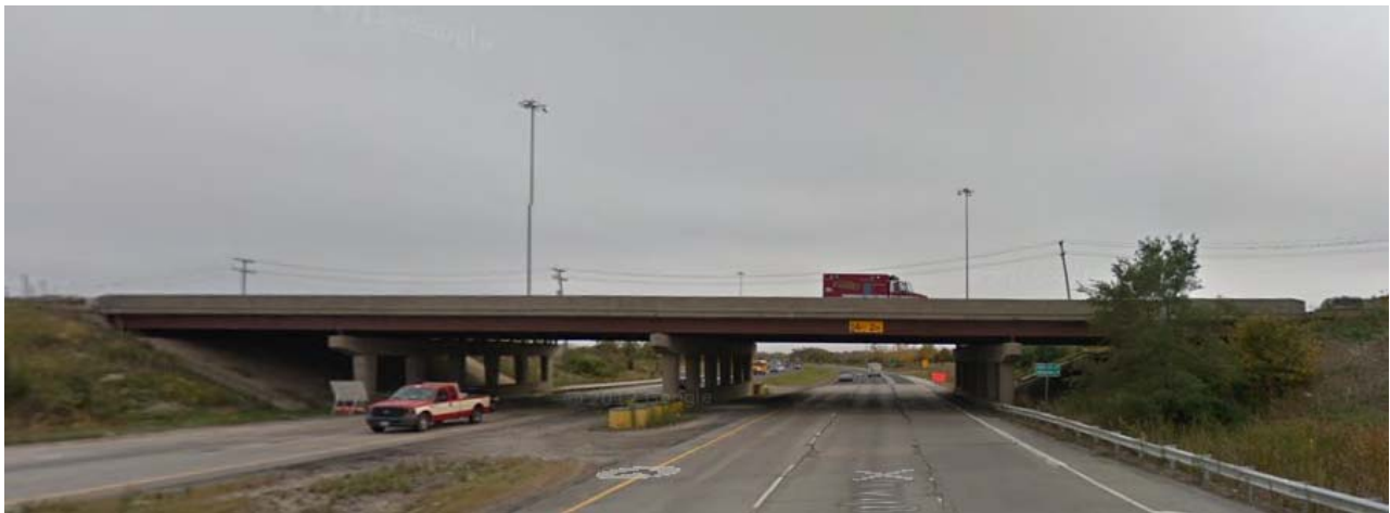
Photo 2: View of IL Rte 120 Bridge over US Rte 41, facing south.
