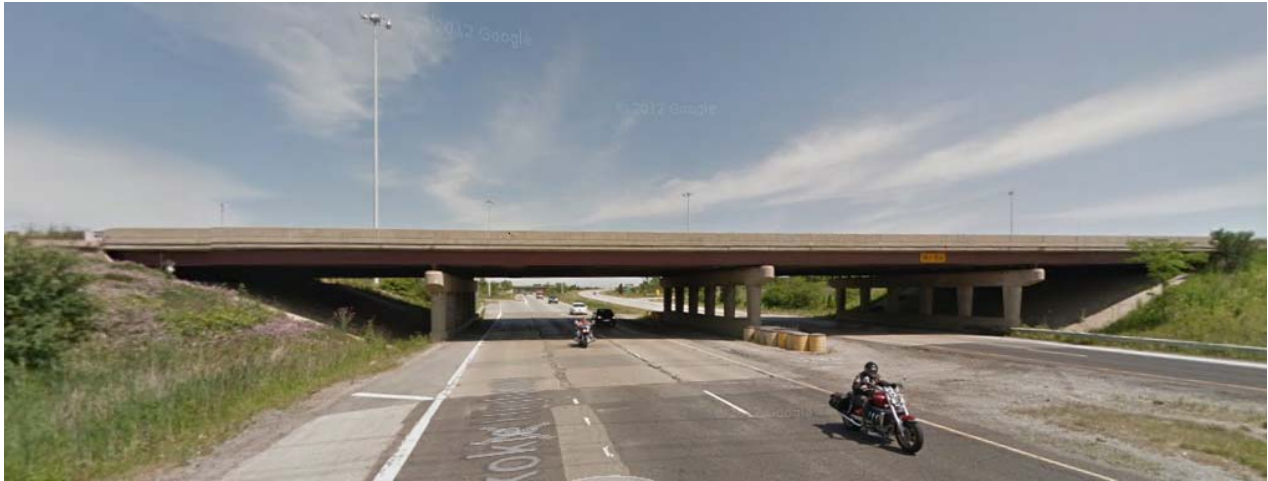
Photo 1: View of IL Rte 120 Bridge over US Rte 41, facing north.
