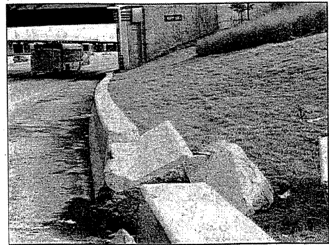
FULL DEPTH BARRIER REPAIR FOR MORE DETAILS SEE SHEET # 8
