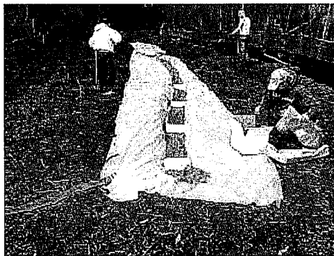
4) Place Flocc Logs (upstream end)
