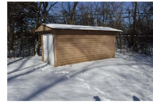
SHED (TO BE REMOVED)
