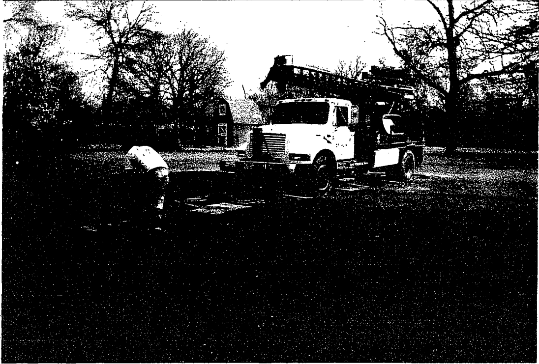
Photo No. 3 - Rig being moved on grassed areas to reach B-4 after planks were placed along its path
