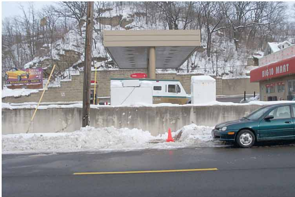
2L. Molo Big 10 Mart (Site 1167-6). Cone marks location of borehole 1167-6b. Photograph taken from south side of Wall Street (foreground), looking north. US 20 is in background, adjacent to retaining wall.
