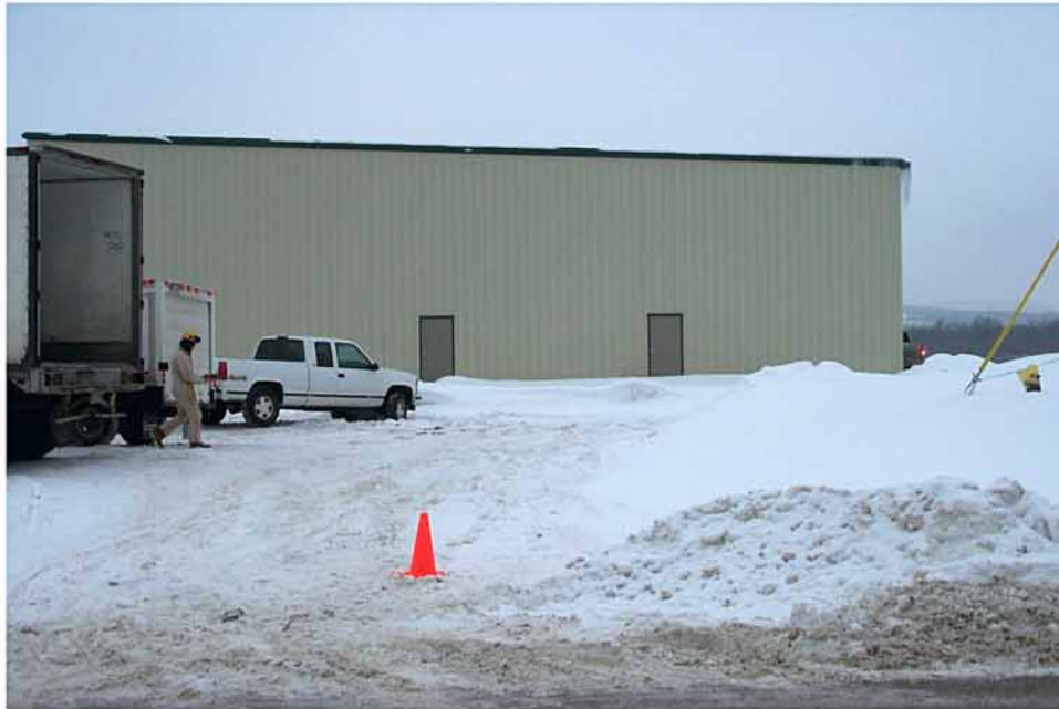
2AA. North Central Farm Lines repair shop (Site 1167-16). Cone marks location of borehole 1167-16a. Photograph taken looking south from US 20 access road (foreground). Northern Illinois Gas Station 290 (Site 1167-15) is at right.
