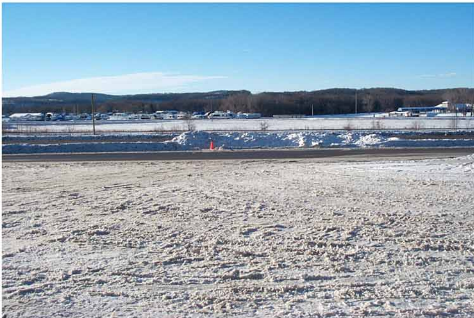
2Z. Ampride gasoline station/Stewart Construction Co. (Site 1167-14). Cone marks location of borehole 1167-14c. Photograph taken looking south from Ampride gasoline station parking lot. US 20 access road is at center of photograph, and US 20 is farther south. Silver Eagle Casino (Site 1167-R) is at far right.
