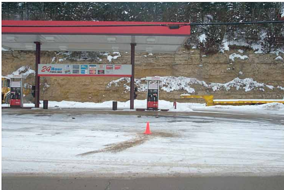
2X. Ampride gasoline station/Stewart Construction Co. (Site 1167-14). Cone marks location of borehole 1167-14a. Photograph taken from US 20 access road (foreground), looking north.
