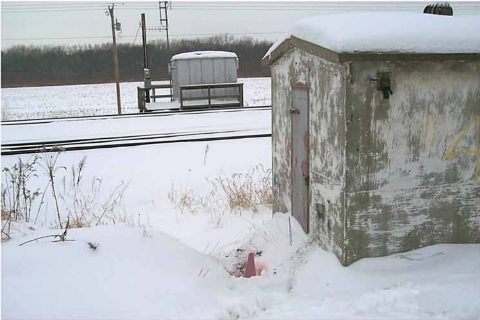
2AC. Burlington Northern Santa Fe Railroad, Murphy Bungalow (part of Site 1167-17). Cone marks location of soil sample 1167-17F. Photograph taken from south of US 20, looking south. New steel bungalow replaced old concrete bungalow.
