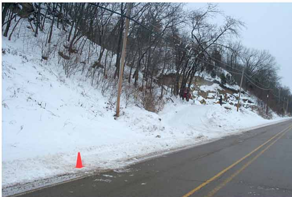
2V. Kieffer Construction storage yard (Site 1167-13). Cone marks location of borehole 1167-13a. Photograph taken from US 20 access road (foreground), looking northeast. Driveway to storage yard is at right.
