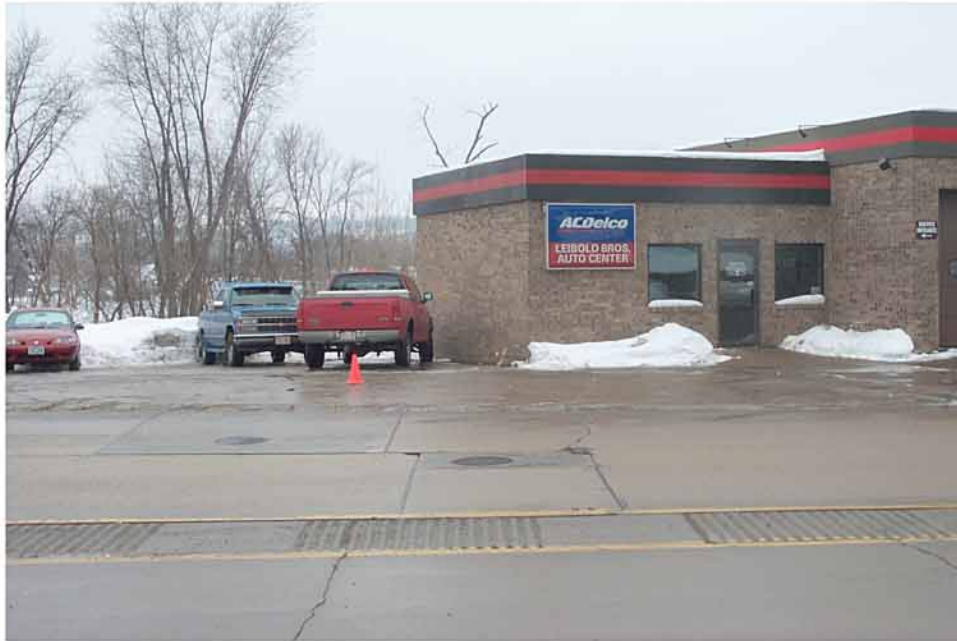
20. Leibold Brothers Auto Center (Site 1167-8). Cone marks location of borehole 1167-8c. Photograph taken from north side of US 20, looking south.
