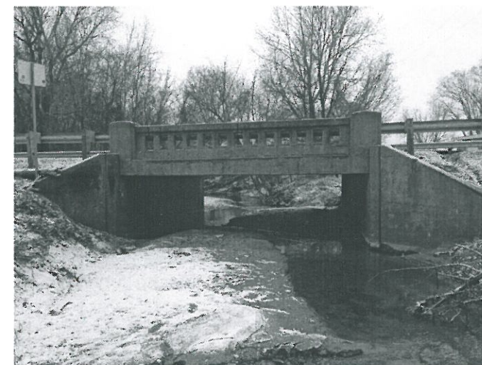
ELEVATION VIEW (7) (Looking West)
