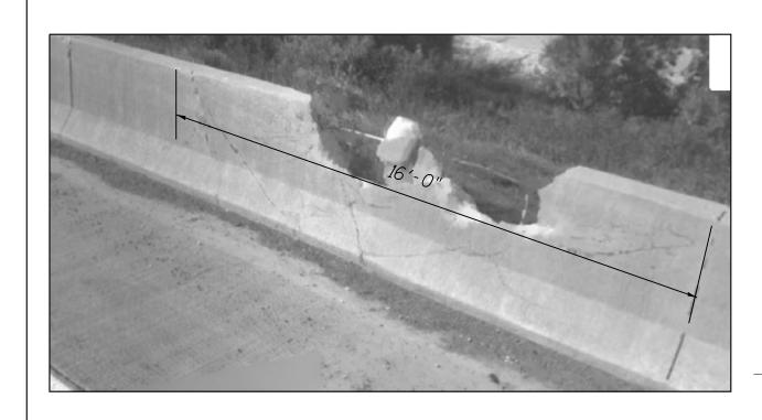
FULL DEPTH REPAIR REPLACE 16' OF BARRIER WALL FOR MORE DETAILS, SEE SHEET #5
