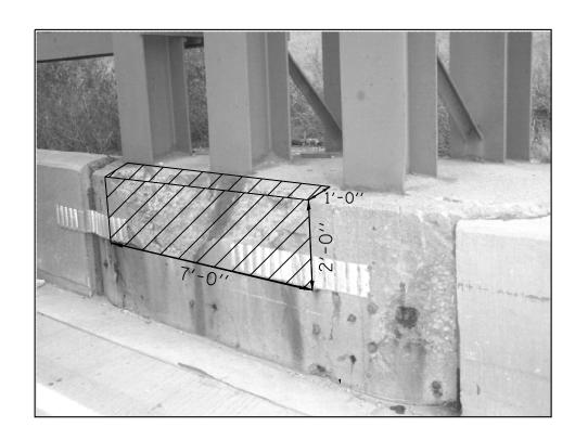
STRUCTURAL REPAIR OF CONCRETE > 5"
