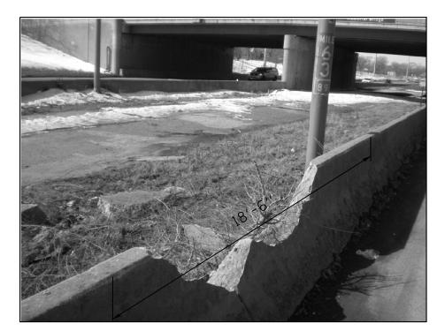
HALF DEPTH REPAIR REPLACE  $18^{1}\!\!/_{2}$  of Barrier Wall FOR MORE DETAILS, SEE SHEET #6
