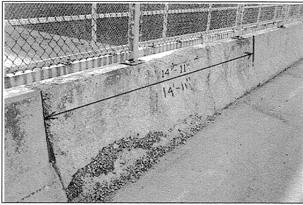
(022-0211) SOUTH PARAPET REPAIR (LOOKING SOUTH) FOR MORE DETAIL SEE SHEET #7
