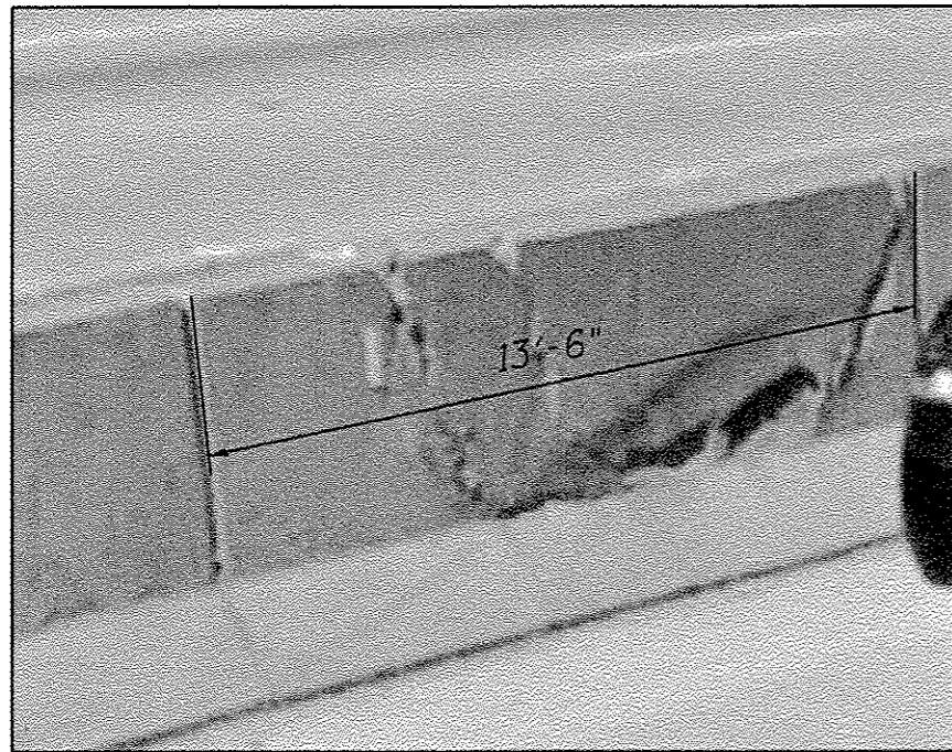
CENTER PARAPET REPAIR FACING NORTHBOUND PARAPET FACE
