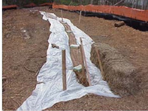
6) Ready for pumping
