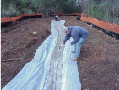
5) Apply Silt Stop (downstream end)
