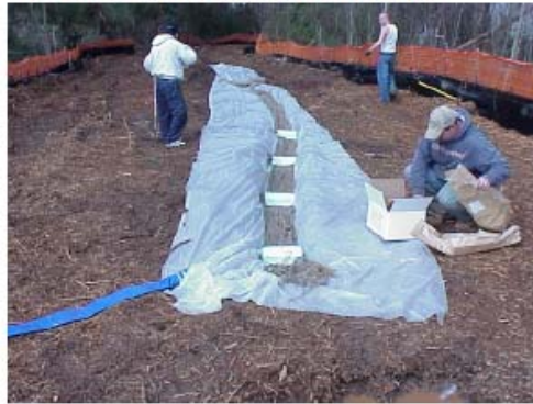
4) Place Floc Logs (upstream end)
