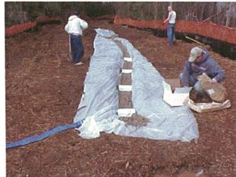
4) Place Floc Logs (upstream end)
