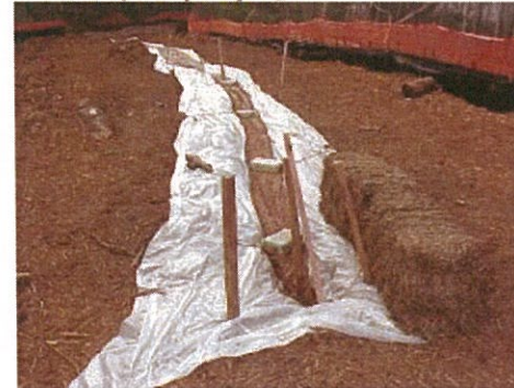
6) Ready for pumping
