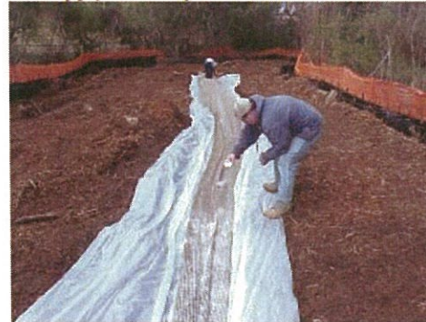
5) Apply Silt Stop (downstream end)
