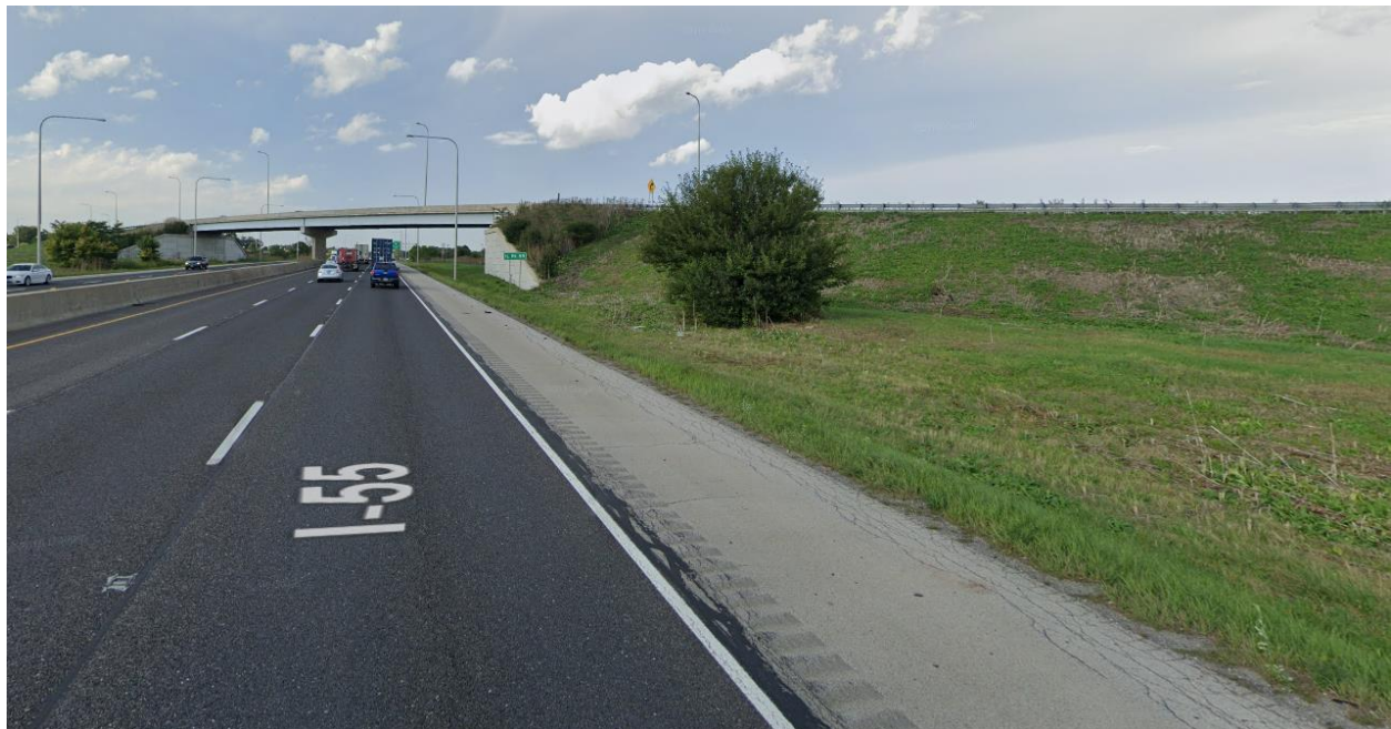
Exhibit 2a – Existing Site Conditions at Proposed East Wall Location, Looking North
