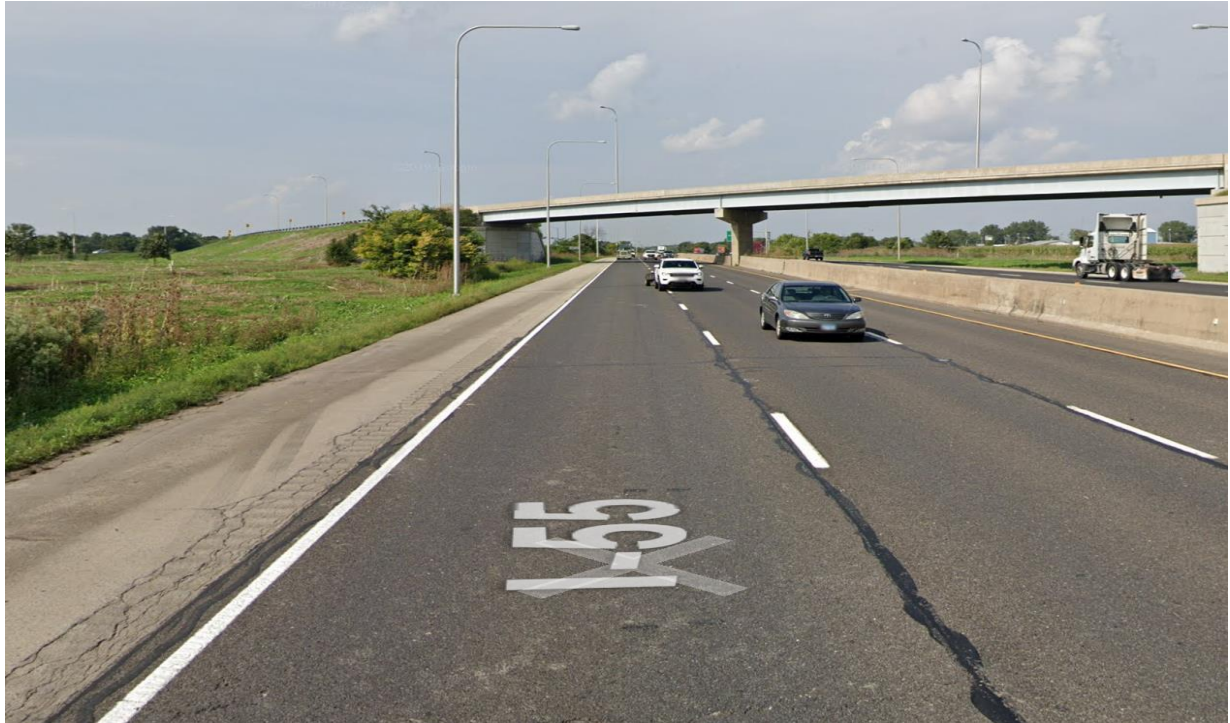
Exhibit 2b – Existing Site Conditions at Proposed West Wall Location, Looking North
