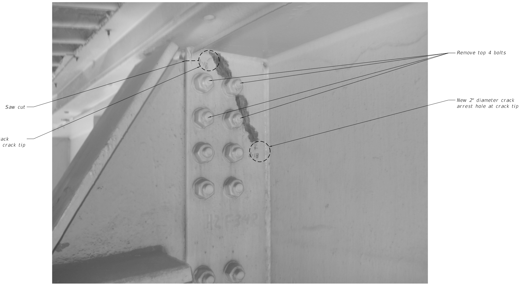
FLOOR BEAM STIFFENER REPAIR Floor Beam 6 at Girder H2
