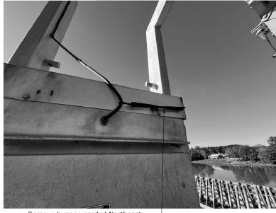
Remove bungee cord at Northeast warning gate and replace with E106. —
