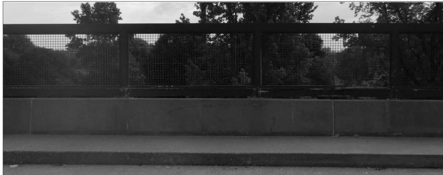
NORTH RAIL - PANEL 11 ①
