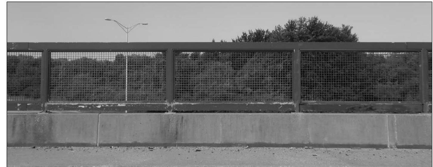
SOUTH RAIL - PANEL 11 ①
