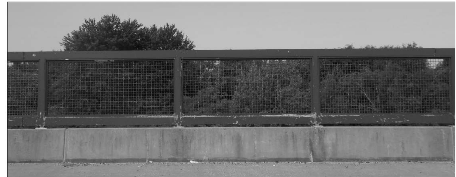
SOUTH RAIL - PANEL 7 ②
