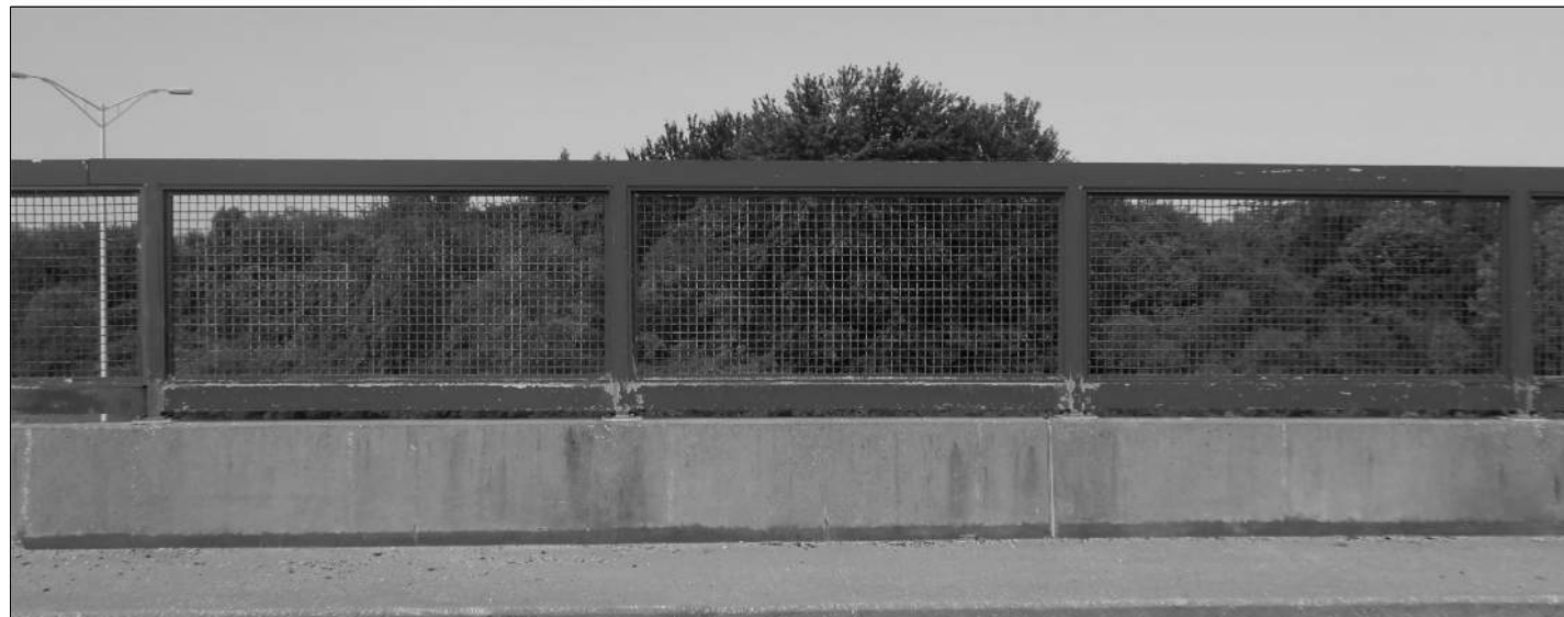
SOUTH RAIL - PANEL 10 ①
