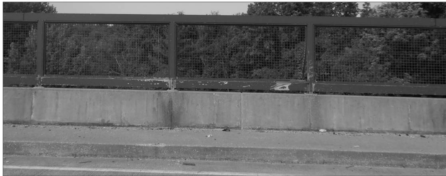
SOUTH RAIL - PANEL 4 ①
