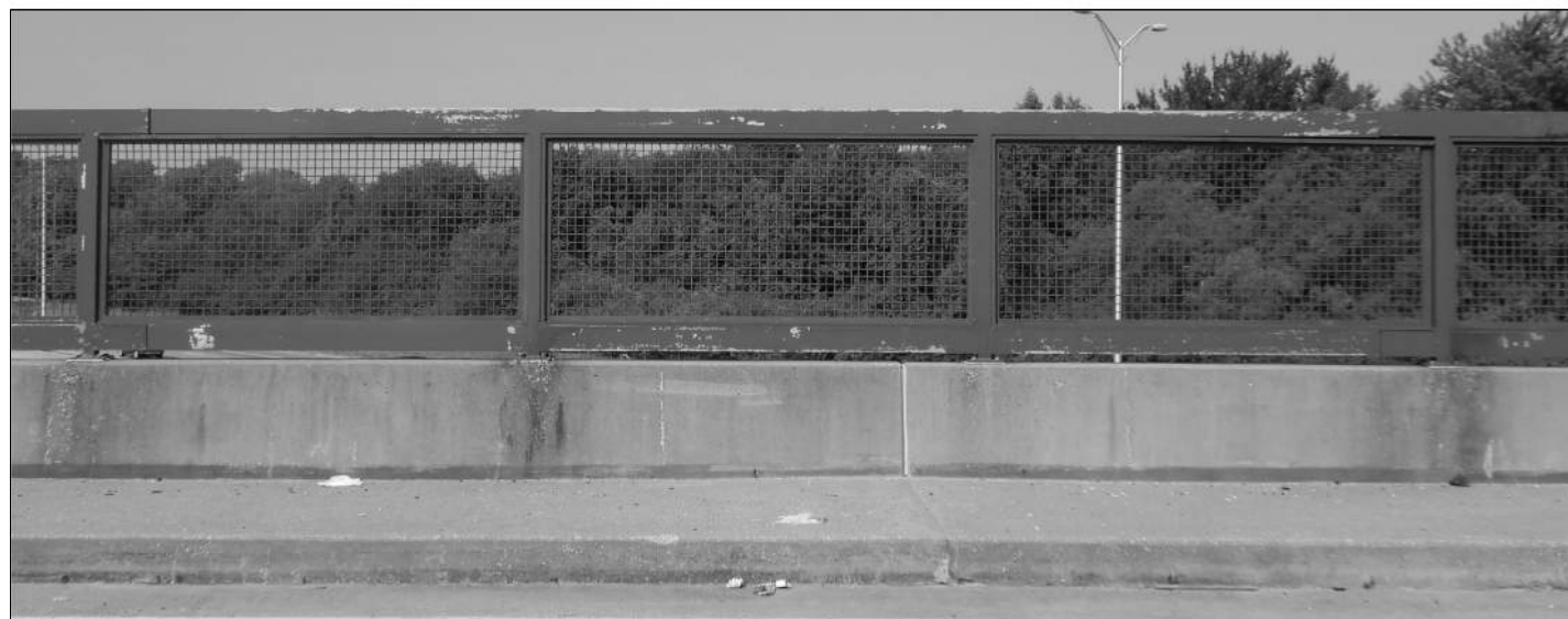
SOUTH RAIL - PANEL 14 ①
