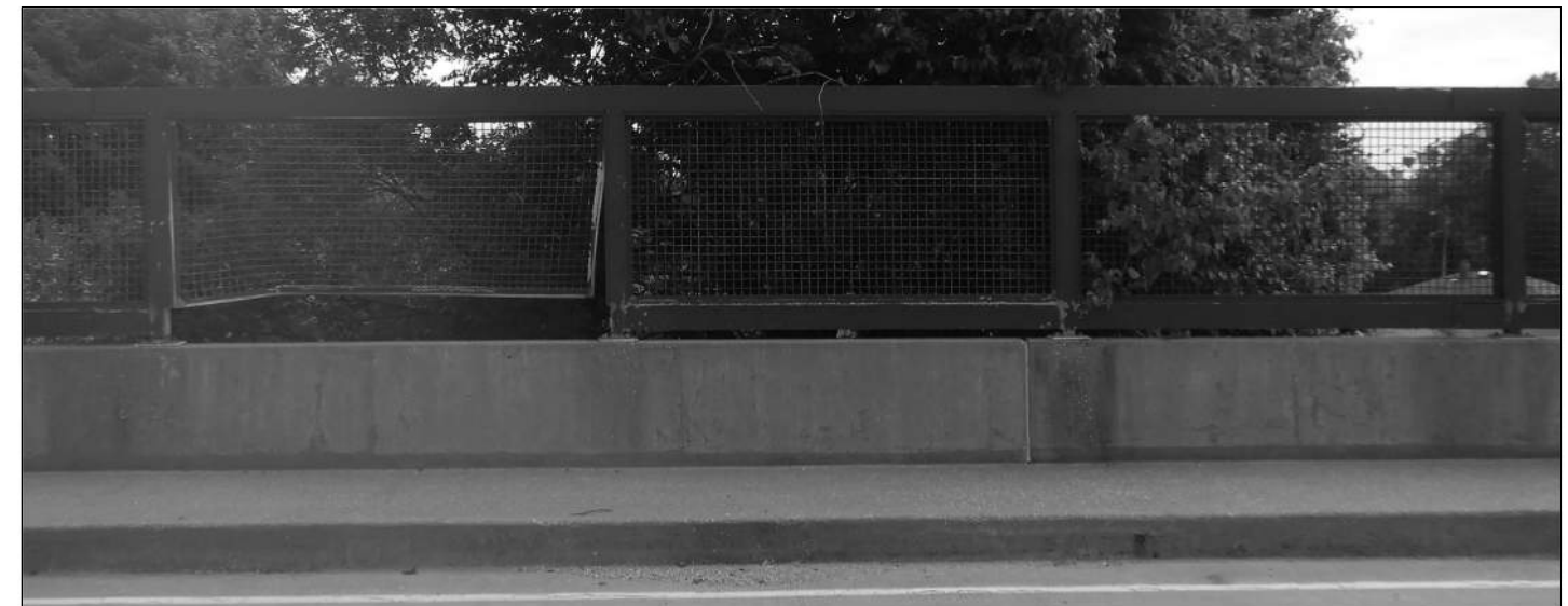
NORTH RAIL - PANEL 16 ①
