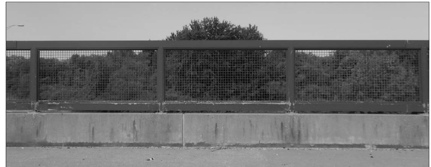
SOUTH RAIL - PANEL 9 ①
