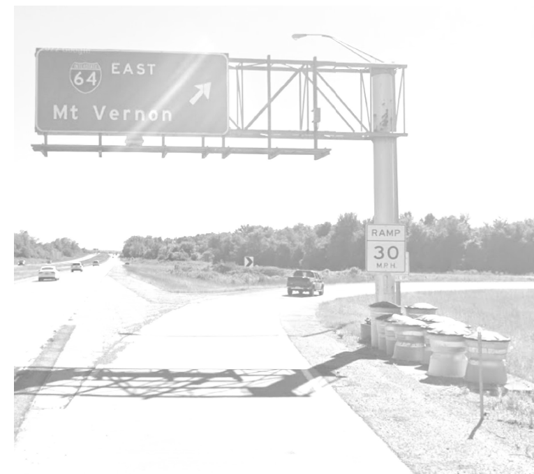
EXISTING SIGNS & TRUSS
