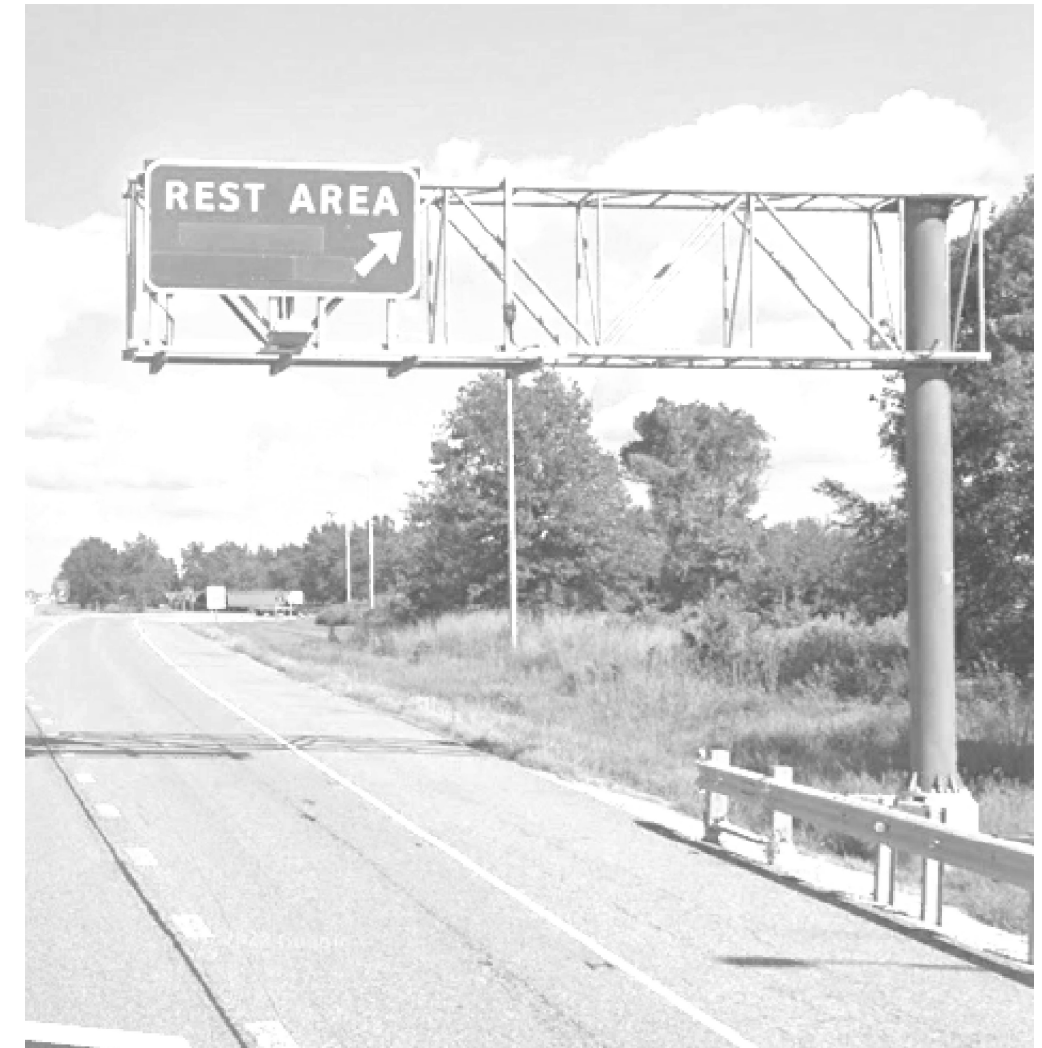
EXISTING SIGNS & TRUSS
