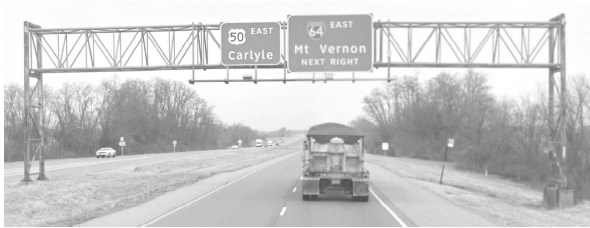
EXISTING SIGNS & TRUSS
