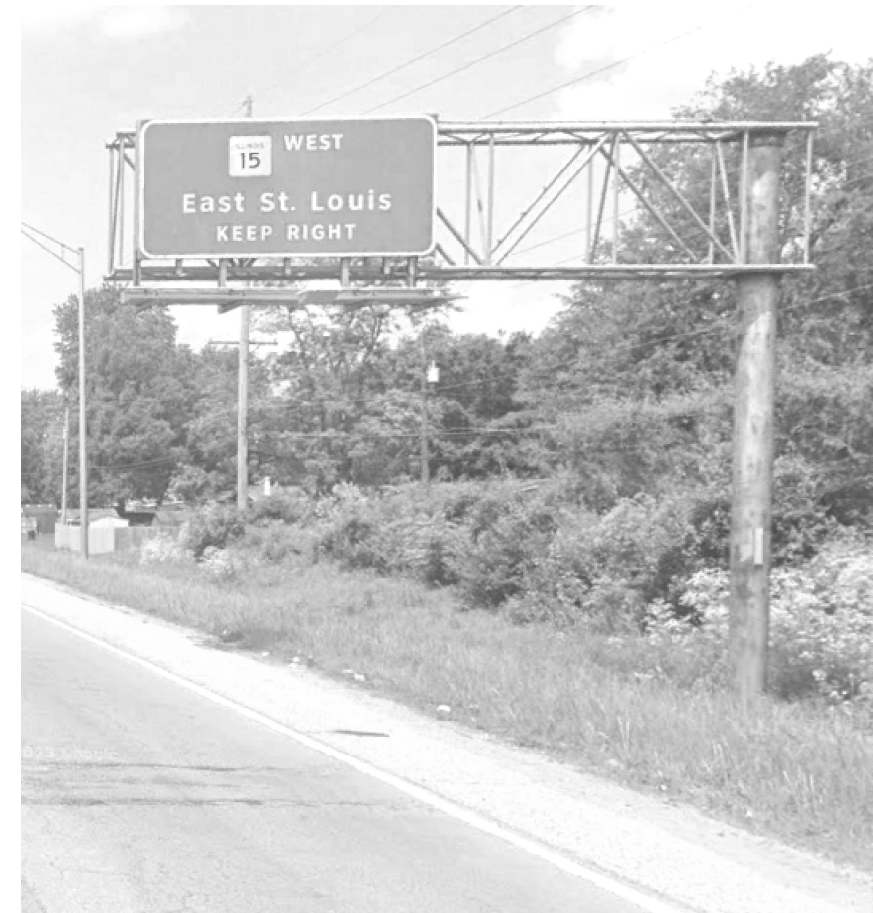
EXISTING SIGNS & TRUSS
