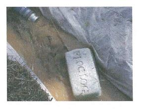
Here is the water being pumped into the treatment ditch. Note the light brown color and turbidity.
