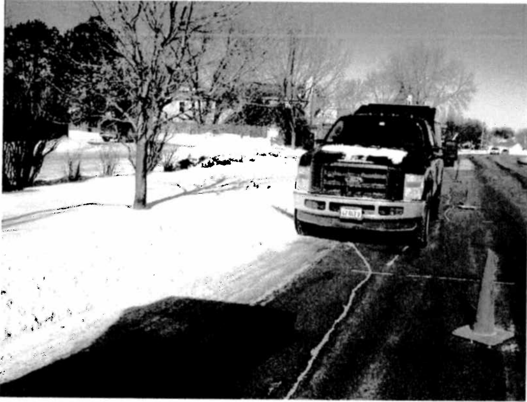
Truck mounted Geoprobe set up at SB-6, view facing north
