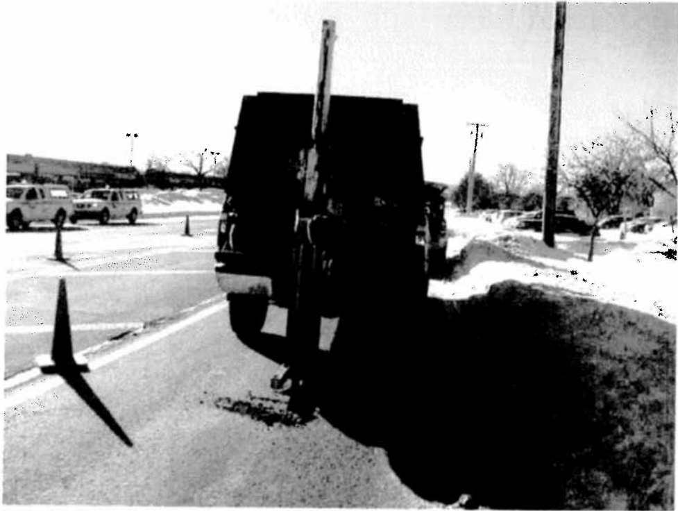
Truck mounted Geoprobe set up at SB-1, view facing south
