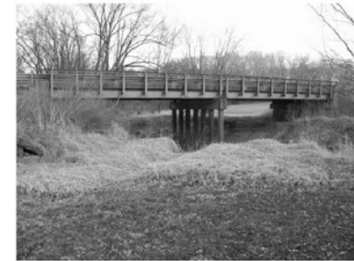
ELEVATION VIEW 3 (Looking East)
