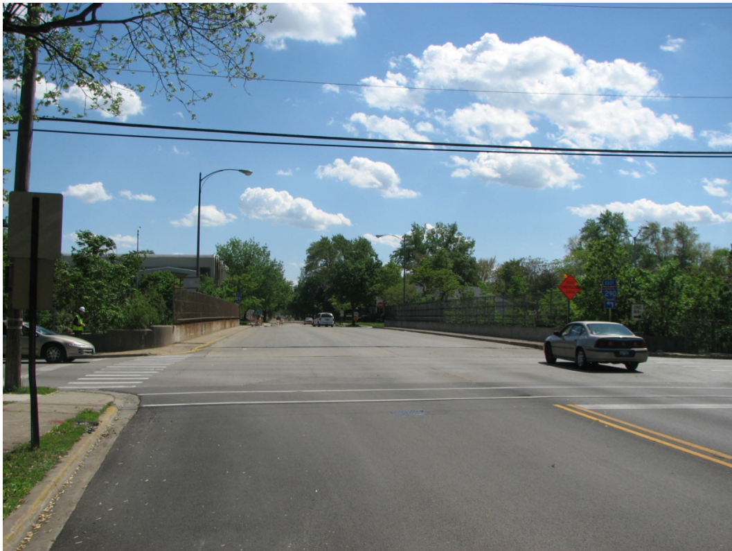
Photo 2 - Top of Bridge Looking South
