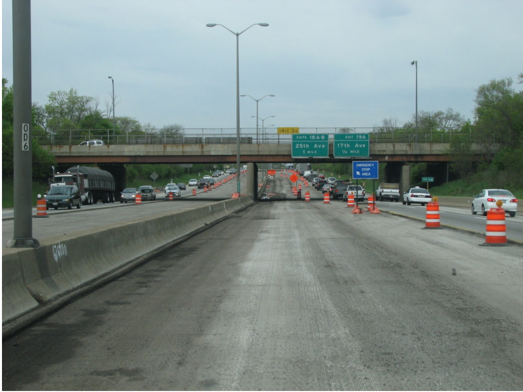
Photo 1 - Overall Looking West
