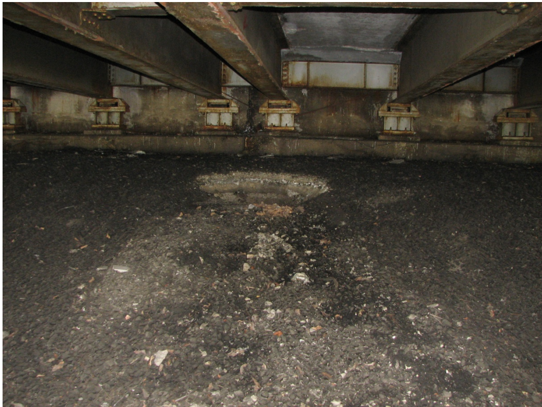
Photo 4 – South Abutment and Slopewall
